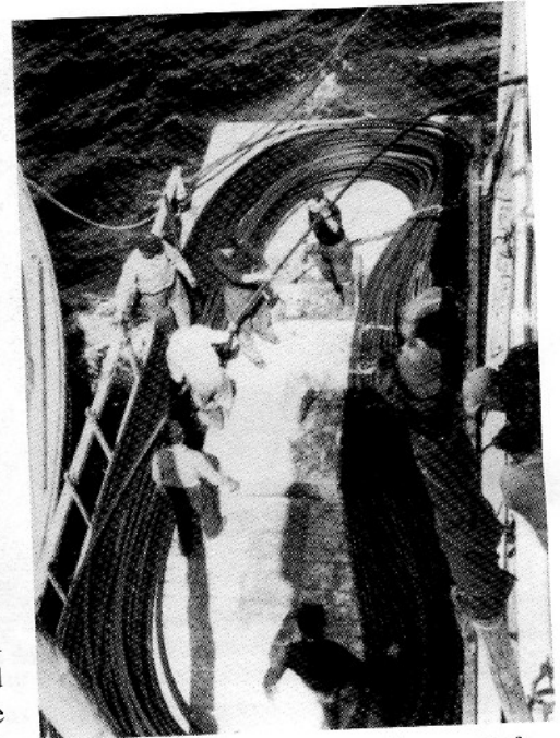
Photo taken in 1949 during replacement of the shore end at Orleans, Cape Cod. Note the cable being loaded on the barge from the Pierre Picard .
